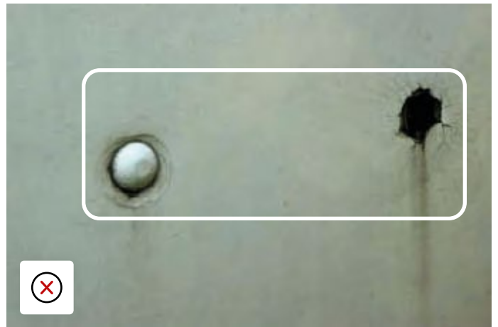
Bolts through GRP side panels.
