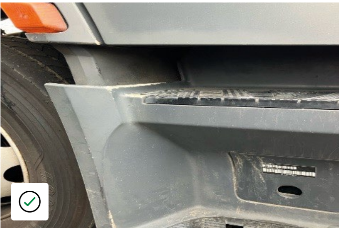
Light scuffing no degradation to the step
