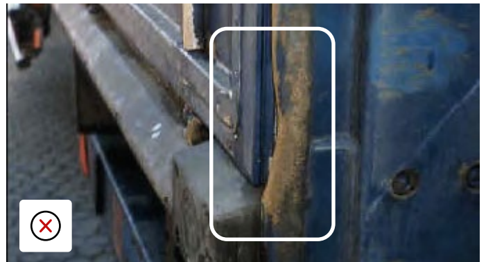
Bent rear door hinge support due to impact, impairing the door operation.
