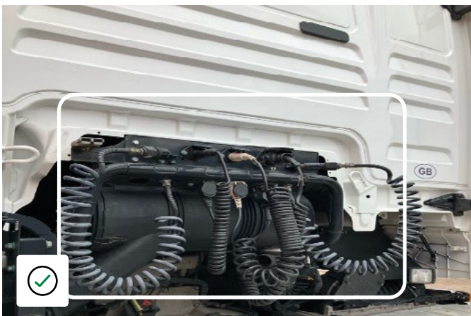
Suzie couplings in good condition & correctly stored
