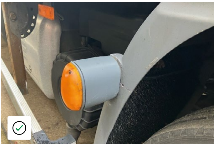
Side repeater & mounting in acceptable condition
