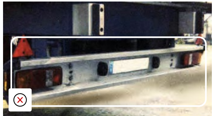
Under run guard bent & requires repair
