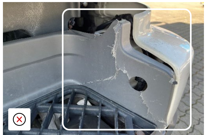
Step support structure unsafe due to impact
