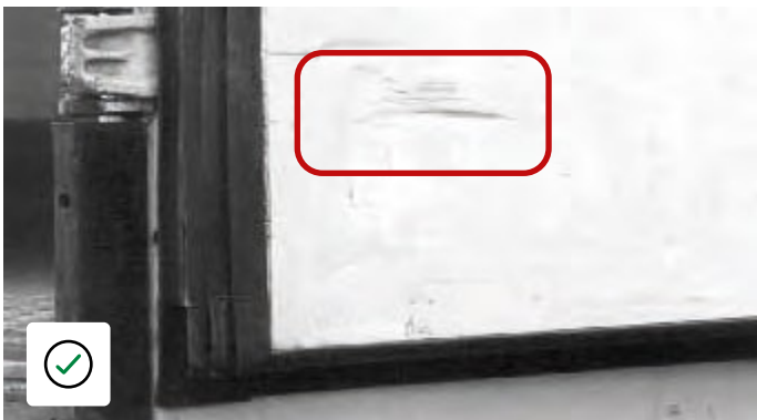
No repair, no recharge to the customer if the inside is not penetrated
